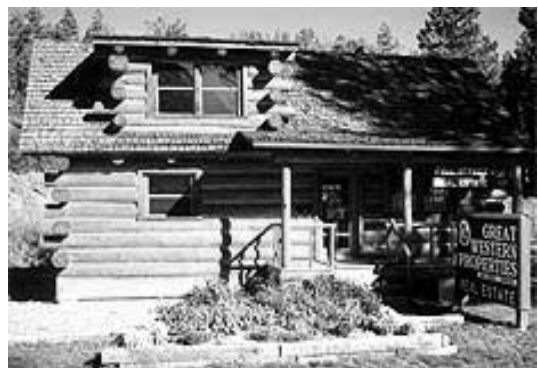
After Corn Cob Blasting
